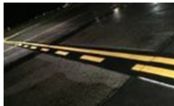
Manoeuvring Area Delimitation Line
