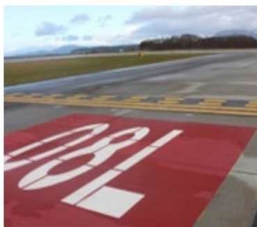
Runway Holding Position Marking
