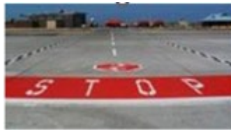
Stop lines/ Markings
